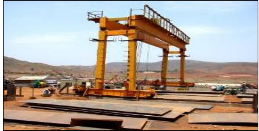
L & T Fabrication Yard : Gantry crane for fabrication – Load test under progress
