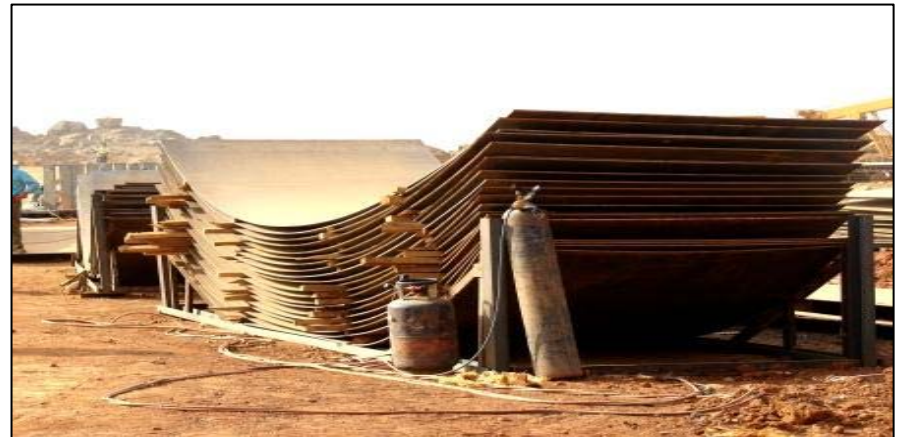
Stock pile of rolled plates for tankages
