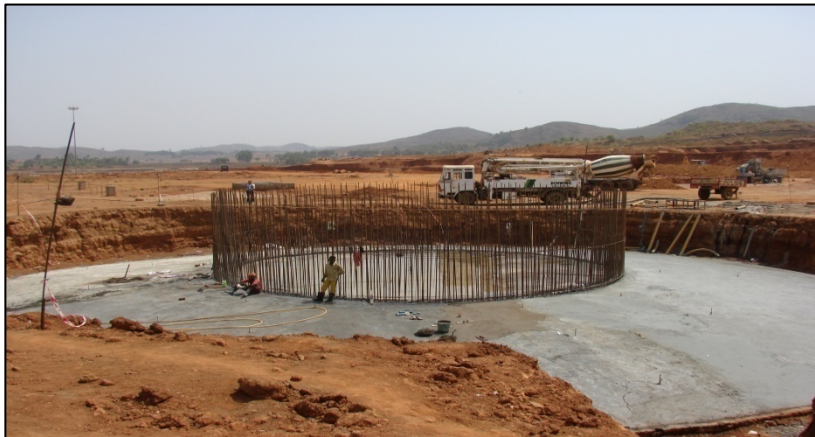
RRCimney for CPP- Raft foundation
